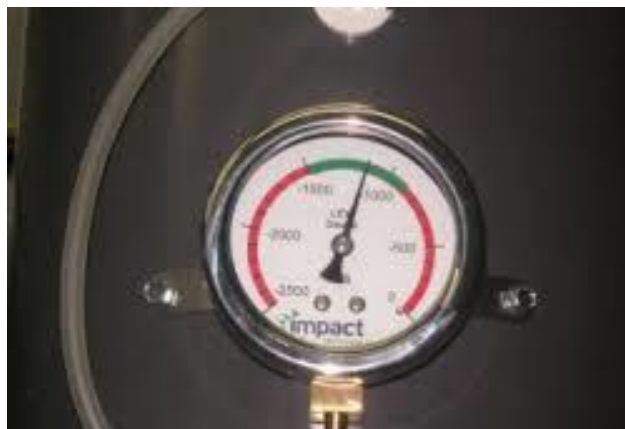
Figure 1 Examples of Colour-coded airflow indicators
