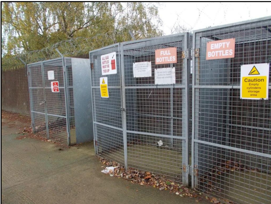
PLATE 2: EMPTY STORAGE CAGES FOR ACETYLENE, ARGOSHEILD AND PROPANE.
