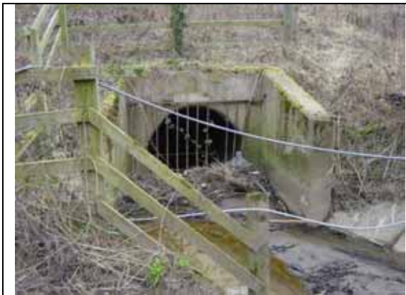
001 Ketley Brook Culvert US Under M54
