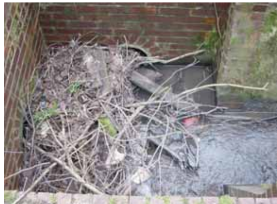
054 Crow Brook US Culvert Sommerfeld Road
