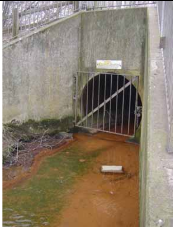
056 Crow Brook DS Culvert Capewell Road Trench Pool Inflow
