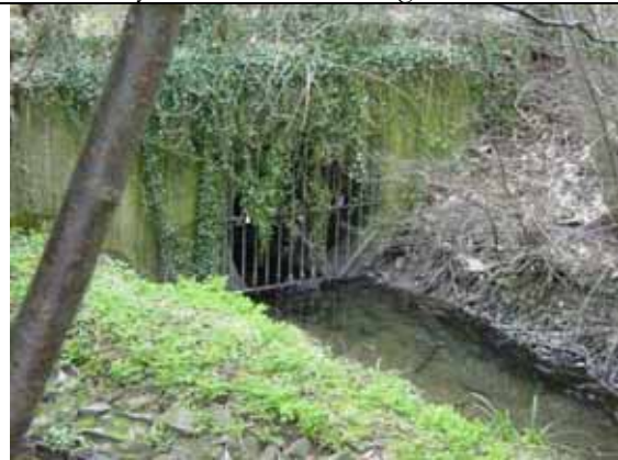
023 Junction of Ketley Book and Hurley Brook Hurley Brook Culvert DS
