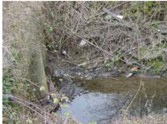
032 Hurley Brook US Culvert A442 Queensway
