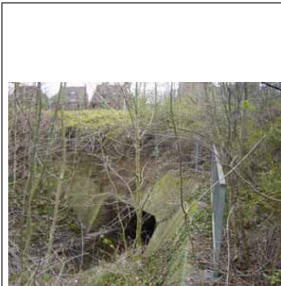
035 Hurley Brook US Culvert Leegate Avenue
