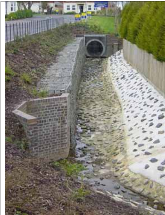
043 Hurley Brook US Limekiln Lane
