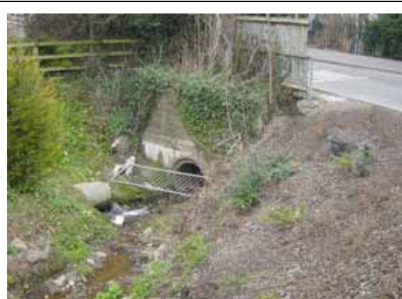
042 Hurley Brook US Culvert Limekiln Lane
