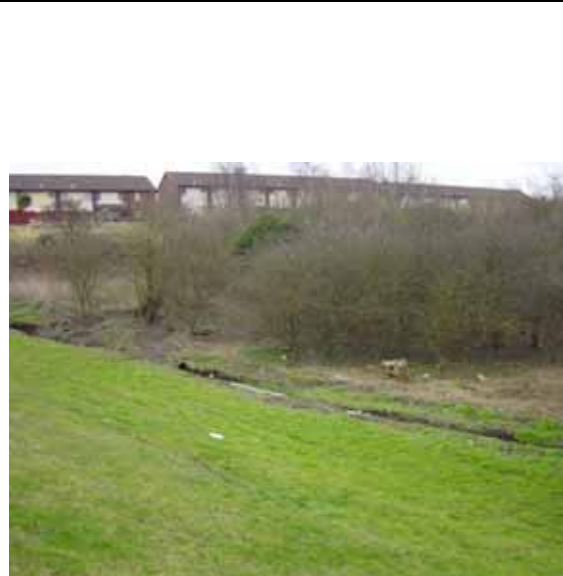
017 Ketley Brook Drain into Sink nr Wedgewood Crescent
