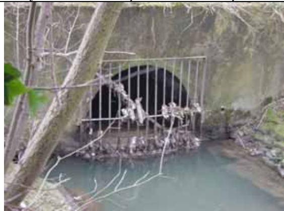
024 Junction of Ketley Book and Hurley Brook Ketley Brook Culvert DS
