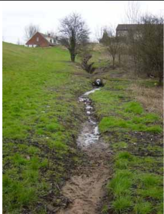
018 Ketley Brook Drain into Sink nr Wedgewood Crescent
