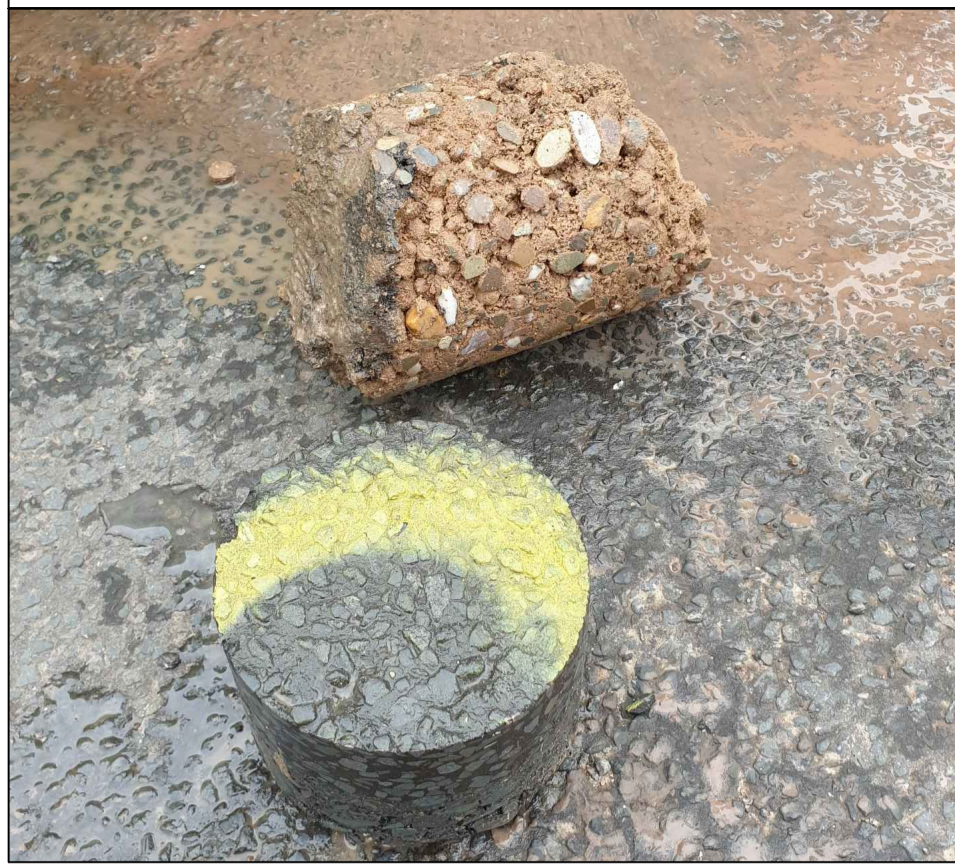
Core 2 @ Chainage 58m: Approx. 100mm Asphalt, 220mm concrete
