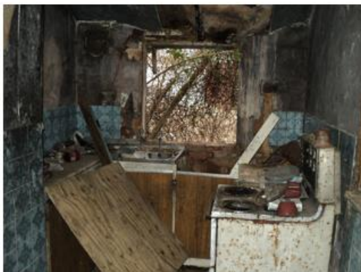
Photos show internal damage by past fire from top of staircase, damage to roof and existing property.
