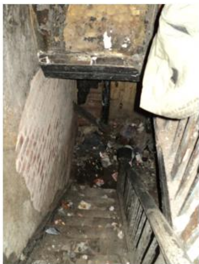
Photos show internal damage by past fire from top of staircase, damage to roof and existing property.
