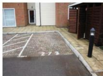
Bin store adjacent to parking space which is not acceptable any parked vehicle will block access to the bin
