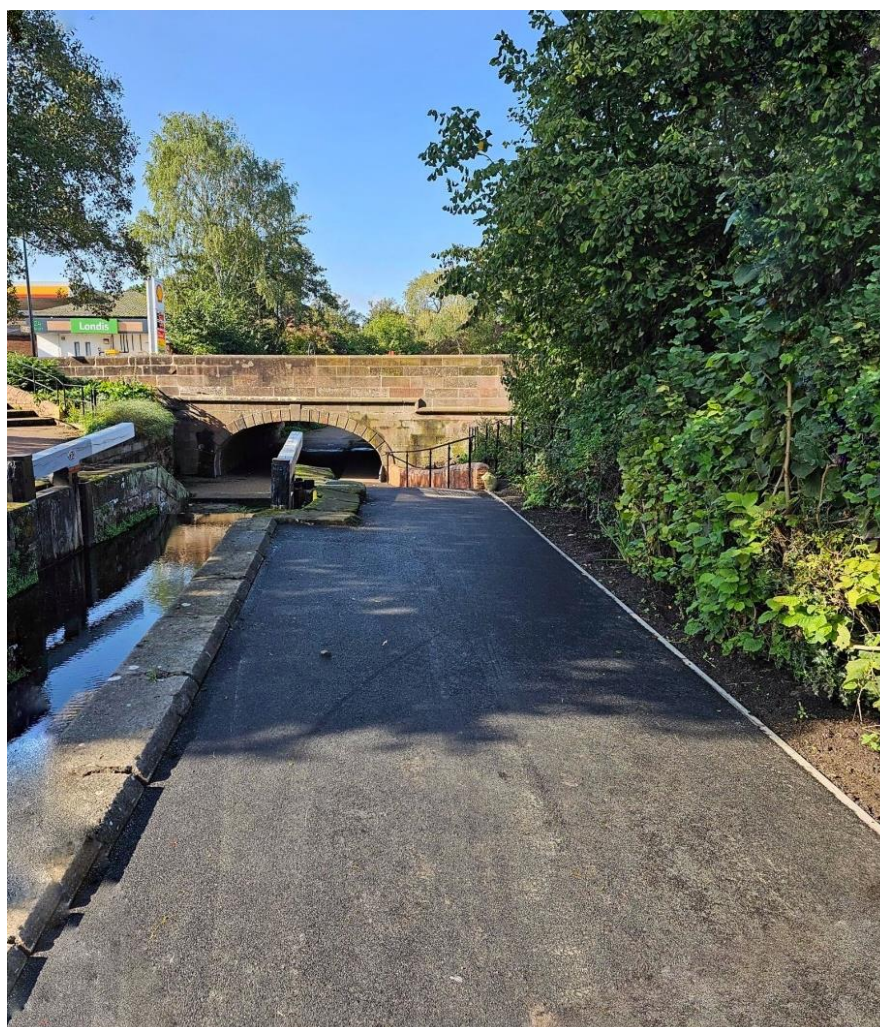
Figure 3: Footpath enhancement alongside Newport Canal
