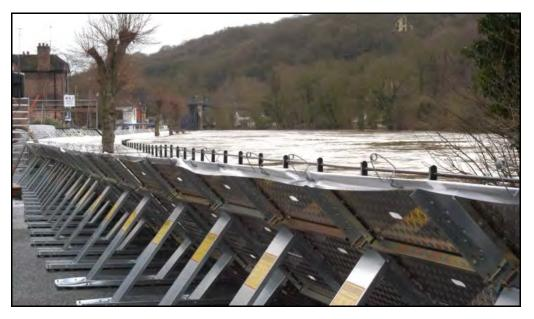
Figure 32 - Barrier Construction
