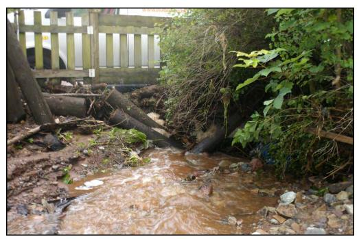
Figure 35 – Blockage of Highway Culvert at Coalport High Street
