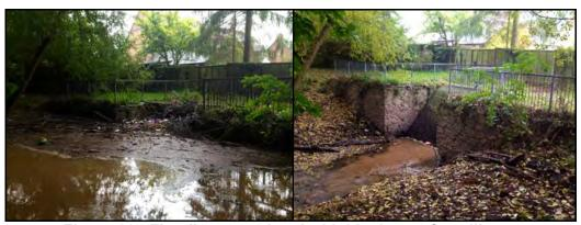
Figure 36 - Flooding associated with blockage of a grille on A culverted watercourse at Bratton
