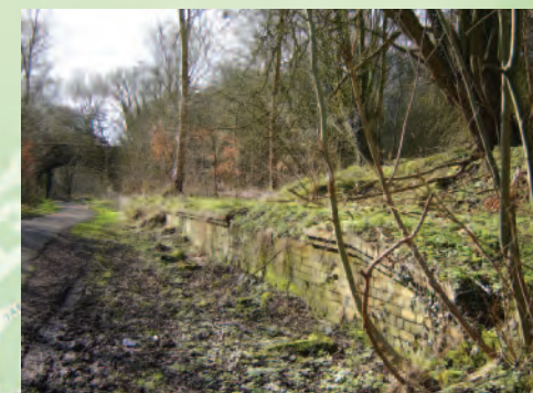
Originally Stirchley Station, renamed Dawley & Stirchley from 9th July 1923. Passenger services withdrawn in May 1952
