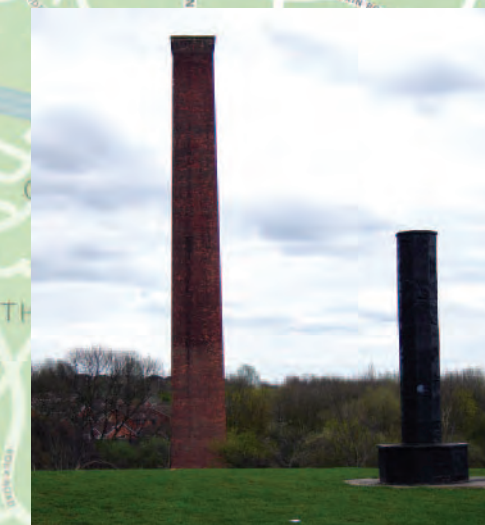
Chimney and Furnace - Built in 1873 by Wellington Iron and Coal Company. Due to bankruptcy in 1877 the furnace was never fired
