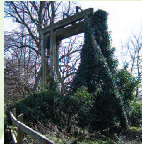
Originally used as part of the Shrewsbury Canal. The canal was built for the use of tub-boats about 20 feet long and 6 feet wide, which were pulled along in trains. The lock was 81 feet long and 6 feet 7 inches wide, which meant that it would hold four tub-boats
