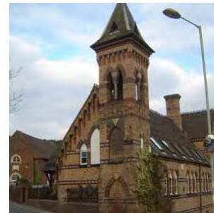
Blue bricks were used for houses as well as public buildings for example 10, Madeley Road, Ironbridge, (left). Polychromatic brickwork acted as a showcase for the local brick trade as seen at Jackfield Church, (centre), and the Wesleyan Infant's School, Madeley Wood, (right).
