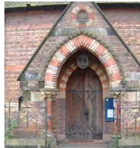
Blue bricks were used for houses as well as public buildings for example 10, Madeley Road, Ironbridge, (left). Polychromatic brickwork acted as a showcase for the local brick trade as seen at Jackfield Church, (centre), and the Wesleyan Infant's School, Madeley Wood, (right).
