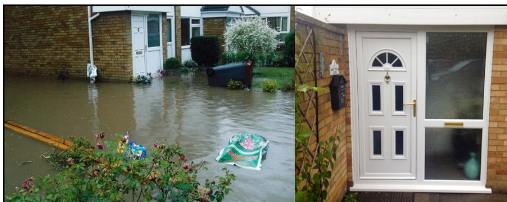
Figure 23 – Example of Benefits from FDGiA Funding in Telford: Provision Flood Resistant Doors to Properties in Wellington
