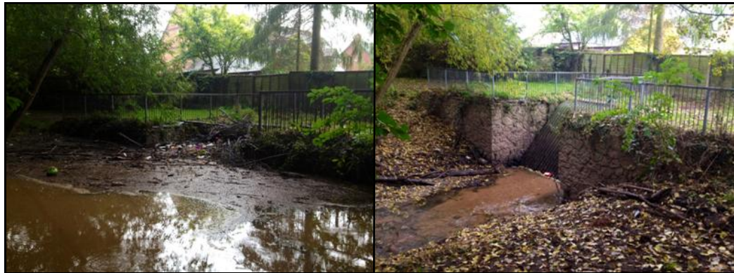
Figure 36 - Flooding associated with blockage of a grille on A culverted watercourse at Bratton
