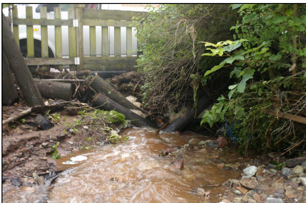
Figure 35 – Blockage of Highway Culvert at Coalport High Street Resulting in the Flooding of 3 Properties
