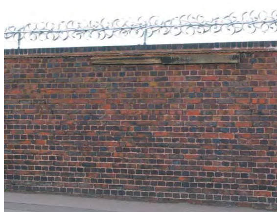
Fig. 33. Cacti anti-scaling device to be used in high risk areas only
