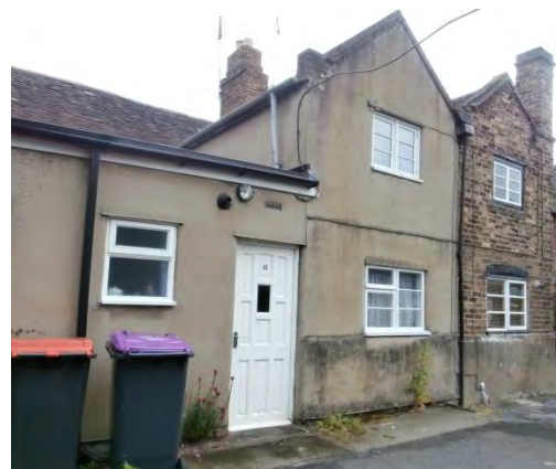
Fig. 26 Inappropriate use of materials and flat roof form for rear extensions on Old Row
