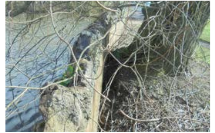
Bulging caused by tree, which was later removed
