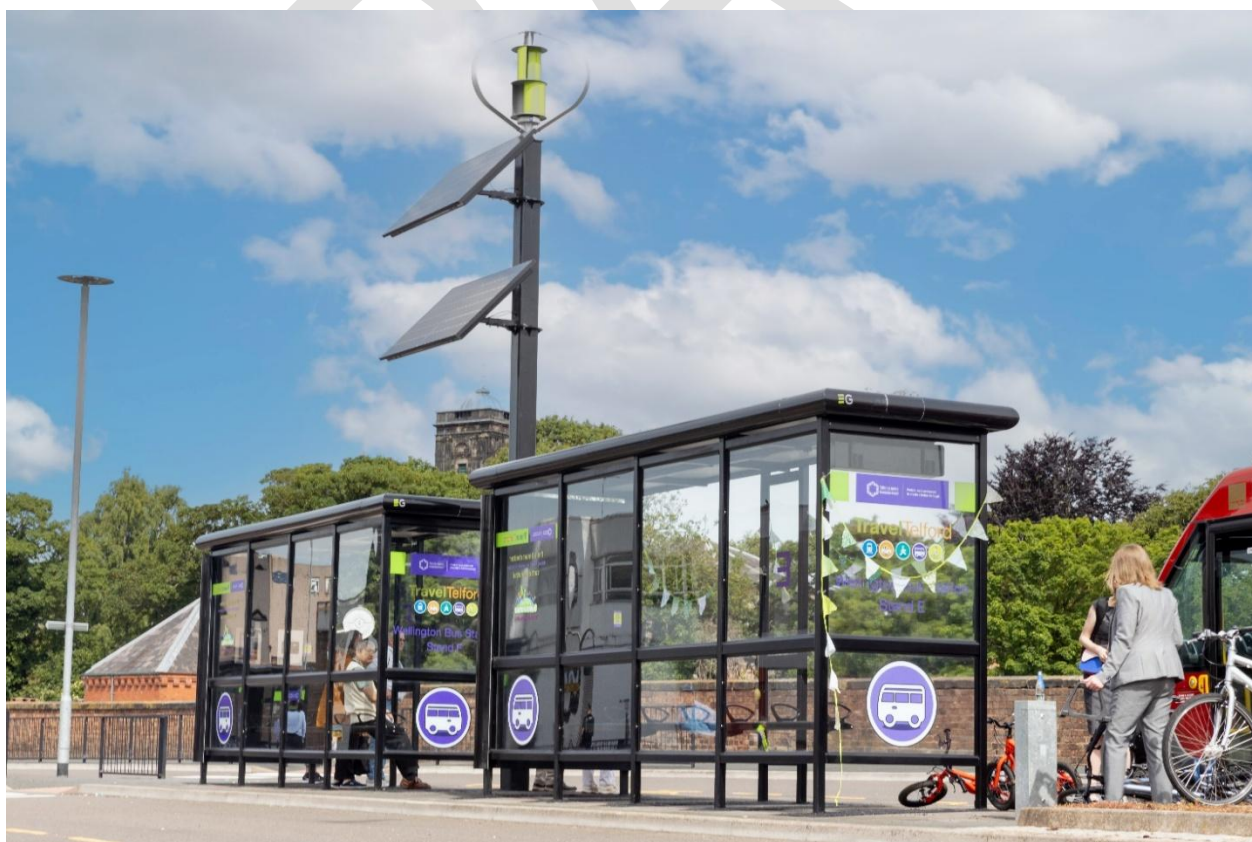
Wellington off-grid bus station
