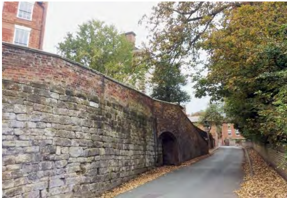
Fig 5.32 Typical brick and stone retaining walls in Coalbrookdale.
