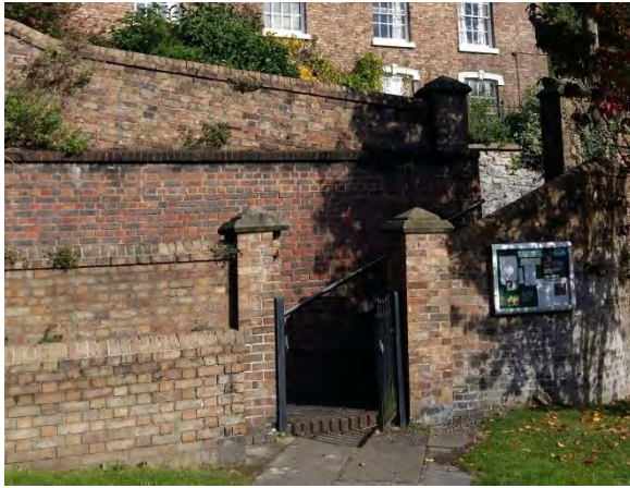
Fig 5.30 Typical brick retaining walls in Coalbrookdale, note the raked brick coursing to the rear wall which follows the slope.
