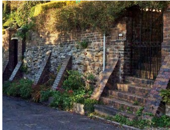
Fig 5.31 Typical brick and stone retaining walls in Coalbrookdale. Subsequent brick buttressing has been added – a traditional solution to strengthening.
