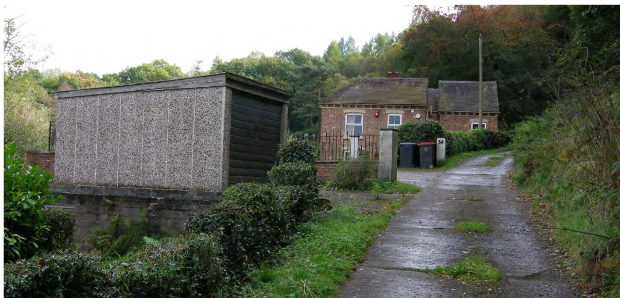
Fig 5.68 In order to create a level area for a garage a platform has been built out over the sloping ground. The garage becomes a very prominent feature in the street scene.
