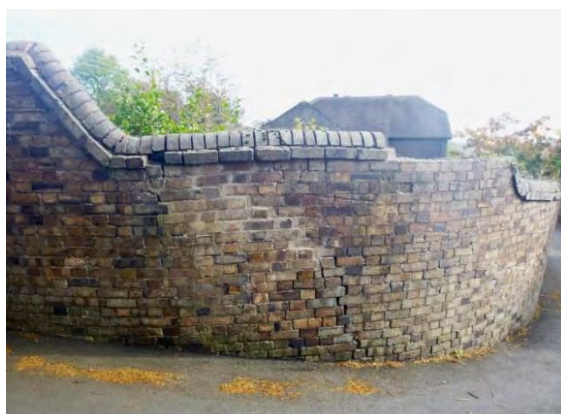
Fig 5.61 The boundary wall on a steep corner bears the scars of many vehicle impacts
