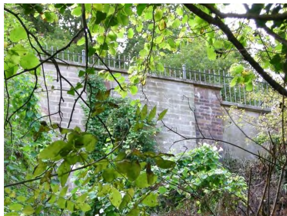
Fig 5.70 Viewed from a footpath below the massive retaining wall, in this case mainly concrete block, becomes a prominent and unattractive feature. Historic retaining walls are a feature of the area but are generally mellow brick or stone.
