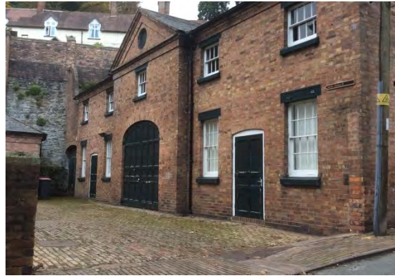
Fig 5.43 Brick paving to Darby House coach and stable yard, Coalbrookdale
