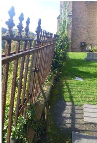
Fig 5.55 St Luke's church - cast iron railings in need of repair, square shafts topped by bold finials on a stone plinth
