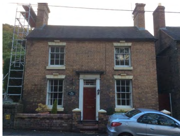
Fig 5.9 Typical small paned sliding sash windows of Georgian character. The meeting rails and glazing bars are very slender and the sashes have no "horns" at the end of the meeting rail.
