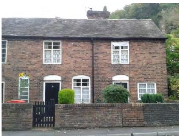
Fig 5.8 Traditional "ladder" casement windows. This example includes iron opening casements. Some traditional ladder windows have timber casements.
