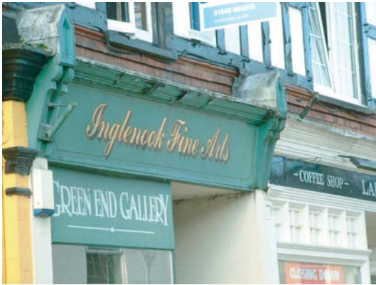
Picture 12 GOOD : Traditional fascia, with cornice above and small architrave below, enclosed with capitals and nicely proportioned sign
