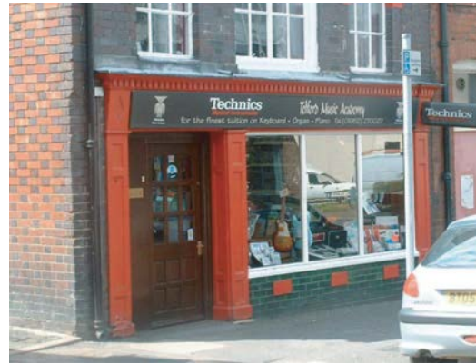
Picture 6 GOOD : Solid recessed panels to the columns, capitals and footings. It creates a solid terminus to the shop front and clear delineation between window and door
