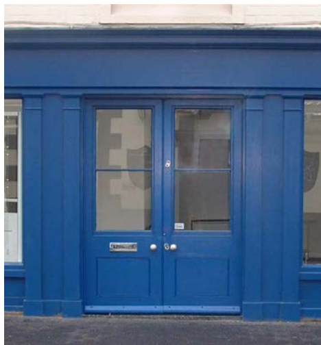
Picture 22 GOOD : Double doors used to create a wide easily accessible entrance
