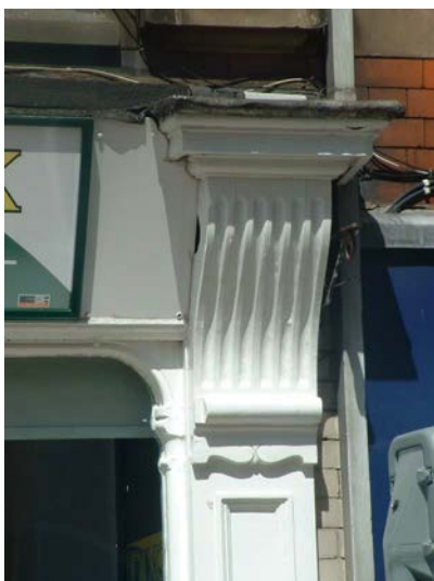
Picture 7 GOOD : Fluted capitals with a cornice at the top to give protection above a recessed moulded column
