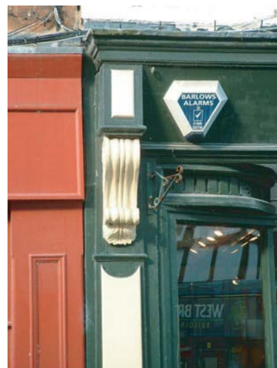
Picture 8 Good : Raised panels on the columns and bracketed capital above contrasting paint
