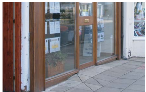
Picture 3 POOR : Stall riser
