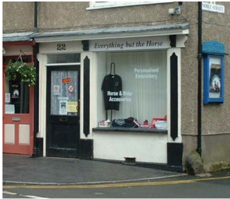
Picture 5 GOOD : Original pilasters with solid footings and moulded panels with bracket capitals to frame the fascia/signboard
